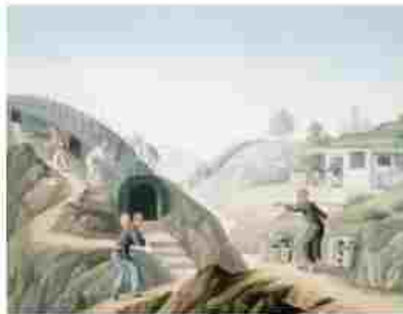
Figure 2.5 Early Chinese porcelain production excelled in reaching high sintering temperatures by use of sloped dragon kiln design, sketched in this early illustration.
